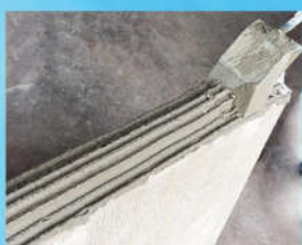
Use toothed trowel to spread mortar
