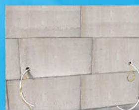
Install pipeline and electric cables easily in hollow cores
