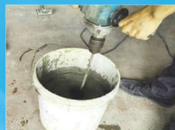
Use ready mixed dry mortar for light block
