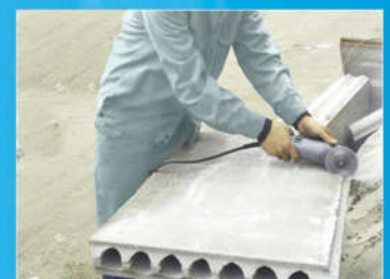
Cut panel by electric hand cutting machine
