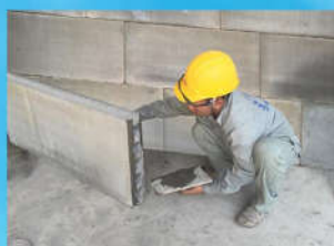
Use flat trowel to apply mortar at the end of panel
